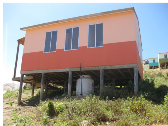
Figure 5: Water tank under houses in Santiago el Pinar.
