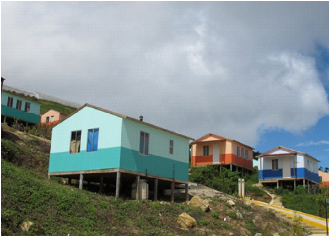
Figure 4.4 Problematic positioning of SRC houses on the steep slope.
